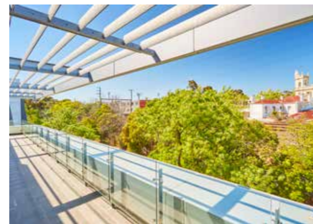
Several outdoor terrace areas
